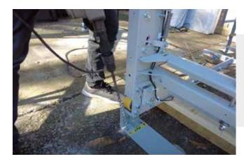
TIP: To gain proper access for the drill, lift the Car Sling, and support with a scrap piece of 2x4.
