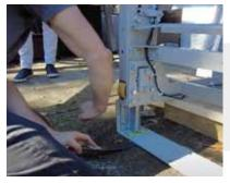
**TIP:** Use a pry bar and a mallet to gently move the rail assembly into the correct position.
